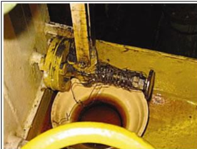
Self-closing gauge glass valve gagged with wire
