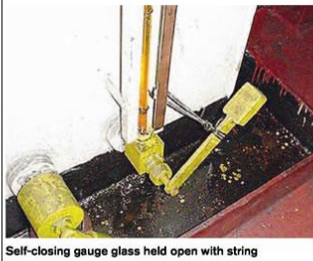
Self-closing gauge glass valve gagged with wire
